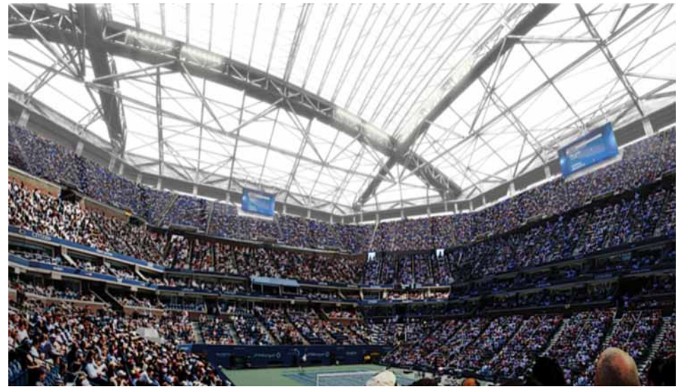
The effort to put a roof on Arthur Ashe Stadium at the National Tennis Center in Flushing, NY was one example of collaboration among various public and private entities.
