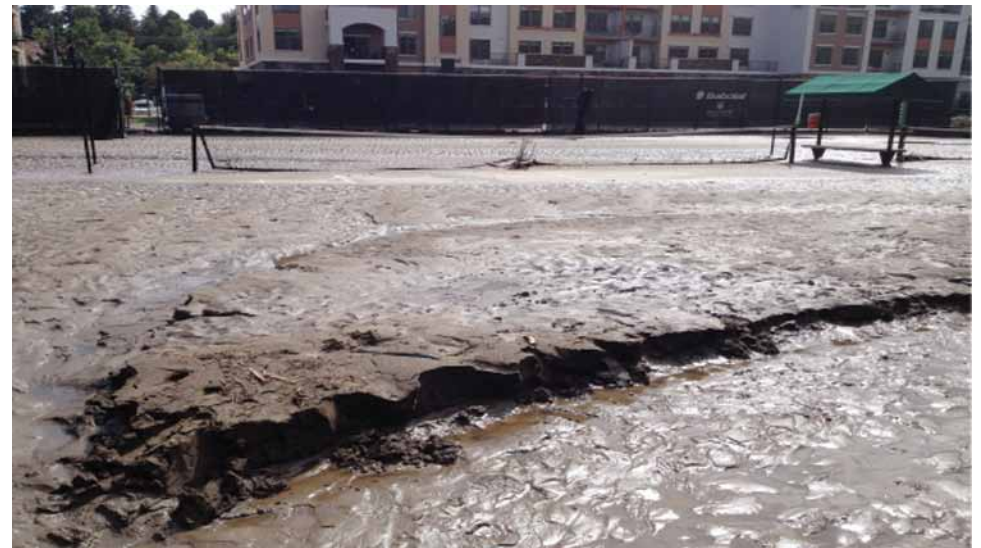
A collaborative effort by the USTA, USTA Intermountain & USTA Colorado helped Rocky Mountain Tennis Center rebuild after the September 2013 Boulder floods destroyed much of the facility.
